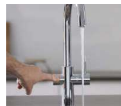
Vent the boiler for 3 minutes via the touch element on the tap.
