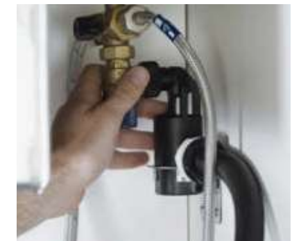
Fix safety group with holder to the cabinet and connect to the filter head outlet.
