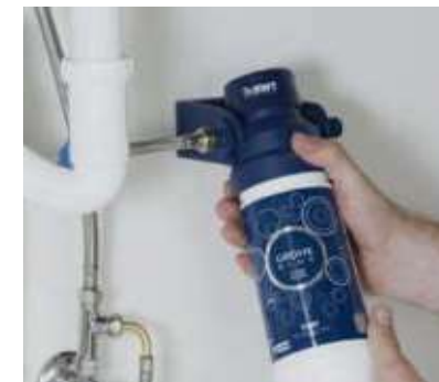
Attach filter holder to the cabinet and screw filter into filter head. Then connect the filter to the cold water supply.
