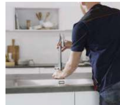
Place tap and mount with fixation set below the cabinet.
