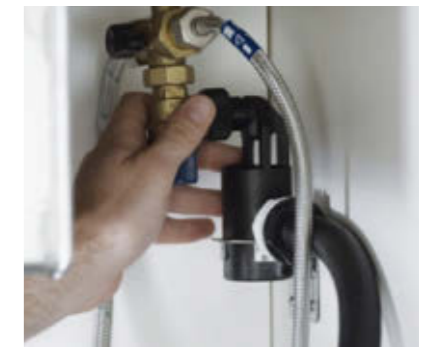
Fix safety group with holder to the cabinet and connect to the filter head outlet.
