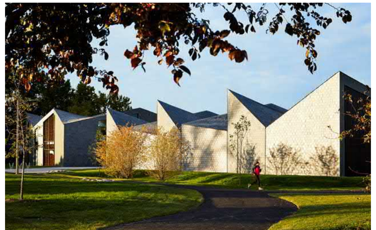
The boathouse comprises two buildings positioned alongside one another in Chicago's new Clark Park.
